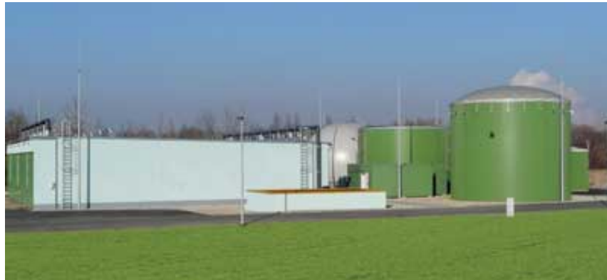
Anaerobic digester facility Source: Harvest Power
